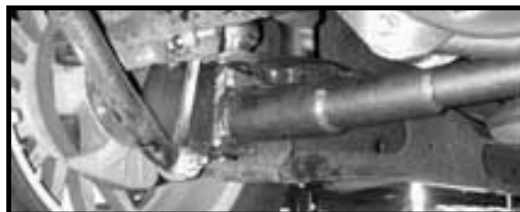
Typical beam installed
