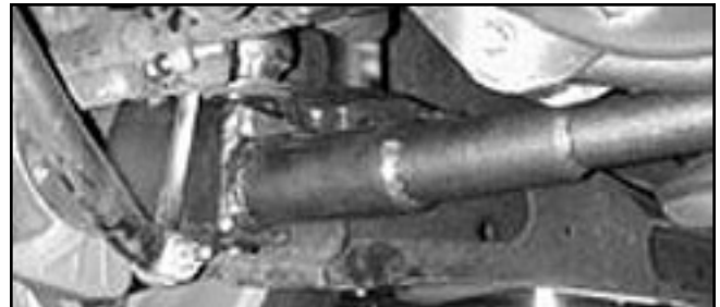
Typical beam installed
