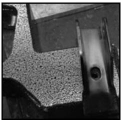
Now after bending the bracket the hole alignment is better but it does not fit flat with the surface of the beam
