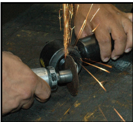
Cut the studs off with a cut off wheel
